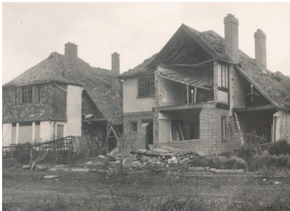
No. 53 Greenway, Hinchley Wood damaged by a VI Flying bomb
